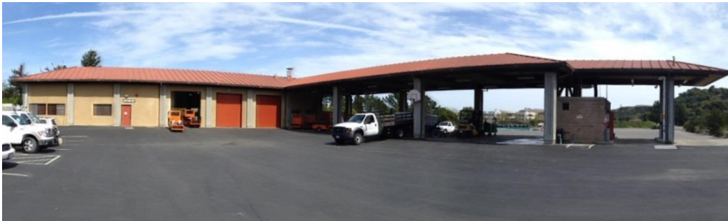
Maintenance Building and Annex
