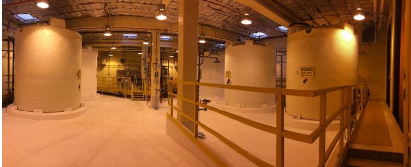
Hypochlorite tanks in storage room
