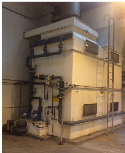
Headworks Odor Scrubber
